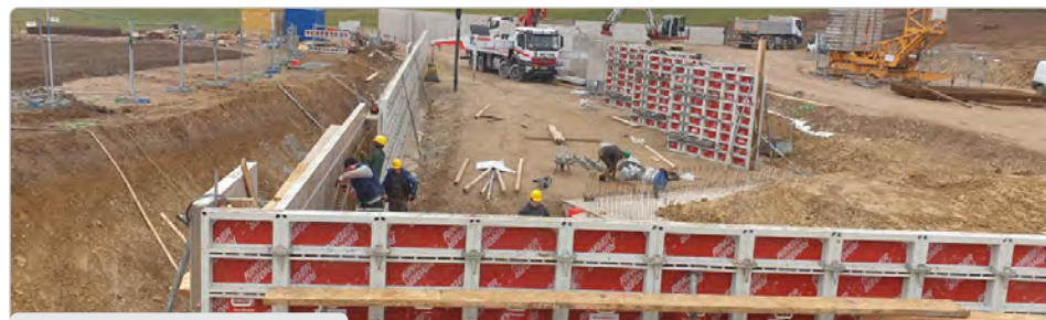
ASZ Lochen in Bau, BAV BR
